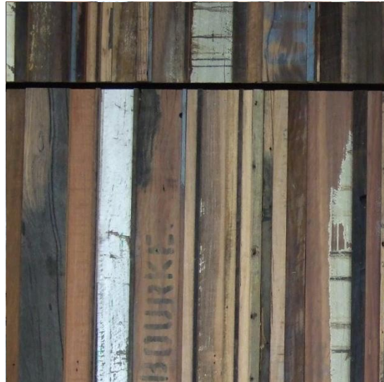
Figure 51: Recycled boards as lining
