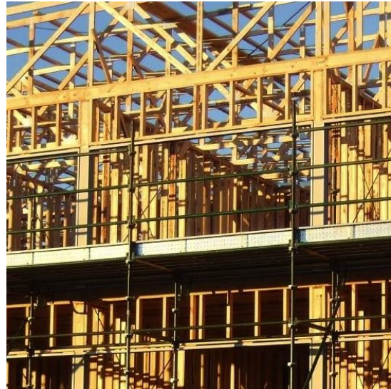
Figure 10: Structural timber frame
