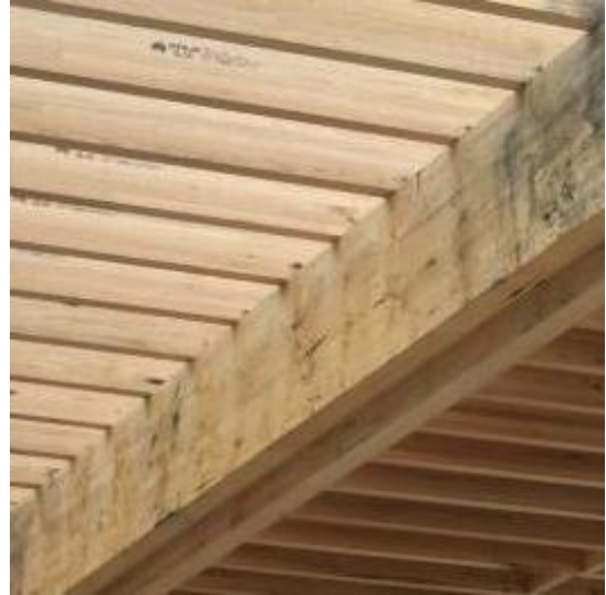
Figure 32: Glulam beams and joists
