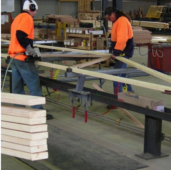
Figure 43: Assembling roof trusses
