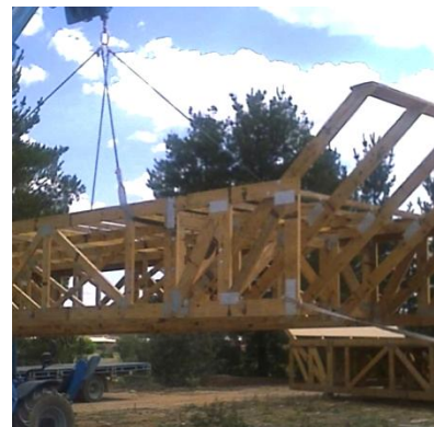
Figure 42: Timber roof module
