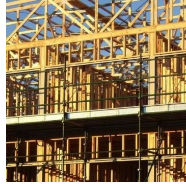
Figure 10: Structural timber frame
