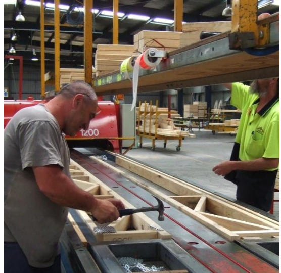
Figure 44: Assembling floor trusses
